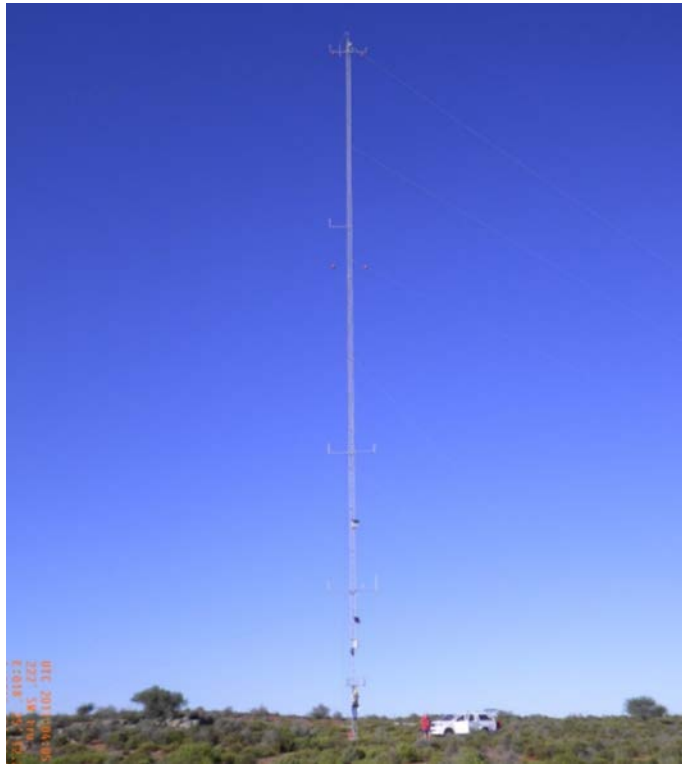
Figure 4.2: Site showing Mast for wind speed at 62m. (Source: WASA station and site description report pg29).
